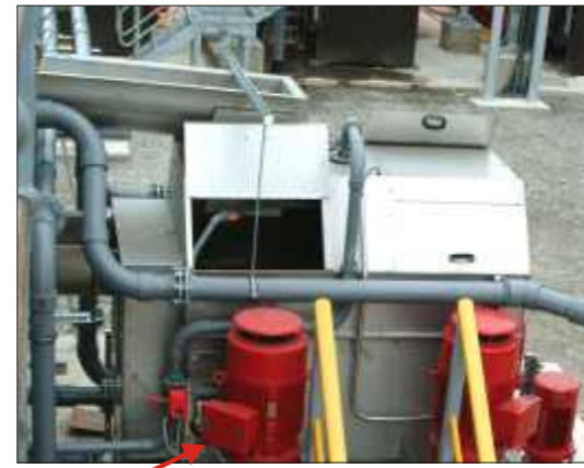
Macipump disintegrates washes and transfers screenings via grit trap.
